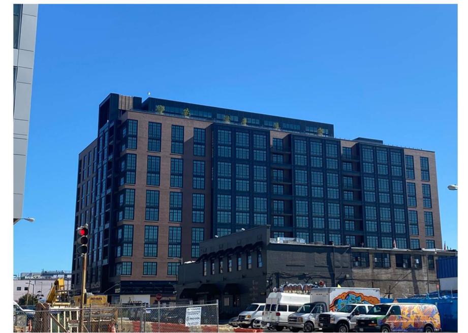
J. Morse St NE & 5th St NE_ 12 Floors Plus Penthouse
